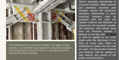
The referenced picture depicts SFRM applied to the gravity load carrying column and primary beams. The BRB's and gusset plates are not part of the gravity load of the structure and are not required to be fire proofed. Although this project was built under the 2013 code cycle, SFRM was still applied to not less than 12 inches for heat transfer, per the approved drawings.
