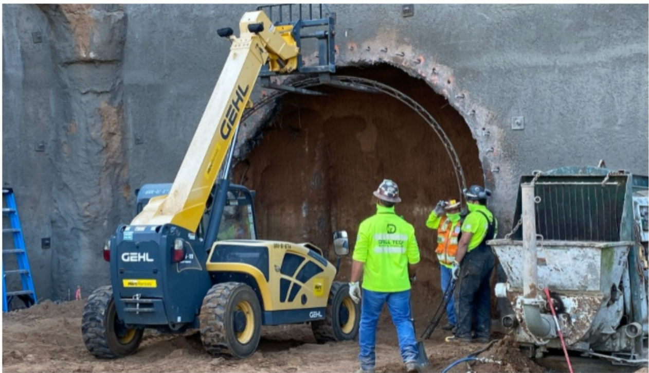
The project team sets the first lattice girder at the entrance of the tunnel. Photo courtesy of Brad Pugh
