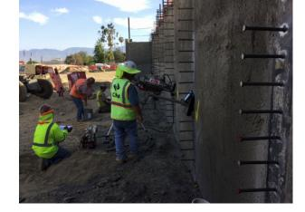
Shoring Tieback Anchor - 200% design load performance test
